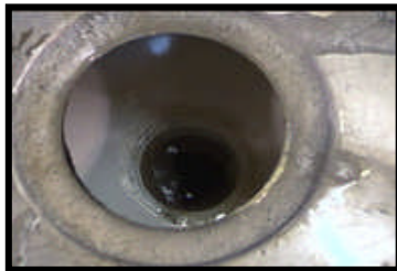
Water level is low when it is below the drain neck.
